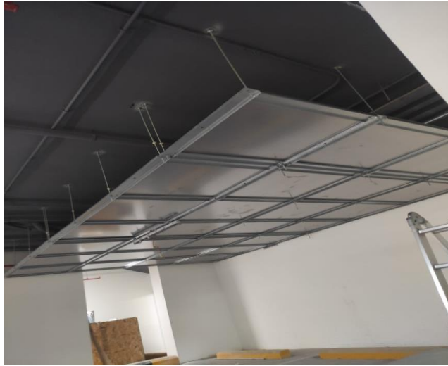
Image 5: Magnetic Shielding Below the MRI Room.
